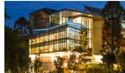
ADVANCED ENGINEERING BUILDING ST LUCIA (UNIVERSITY OF QUEENSLAND), AUSTRALIA
